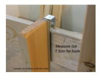
We now have to position the ladder. If the ladder is going on the right handside make a small pencil mark in on the top side rail. The mark should be 7.5cm away from the corner post. This mark now shows you where to position the ladder away from the corner post.
