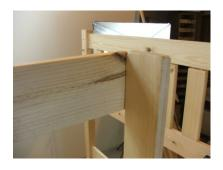
Once the ladder is on place grab the two front guard rails. Start with the first rail and position from the corner post to the top of the ladder strut. Then screw in place.
